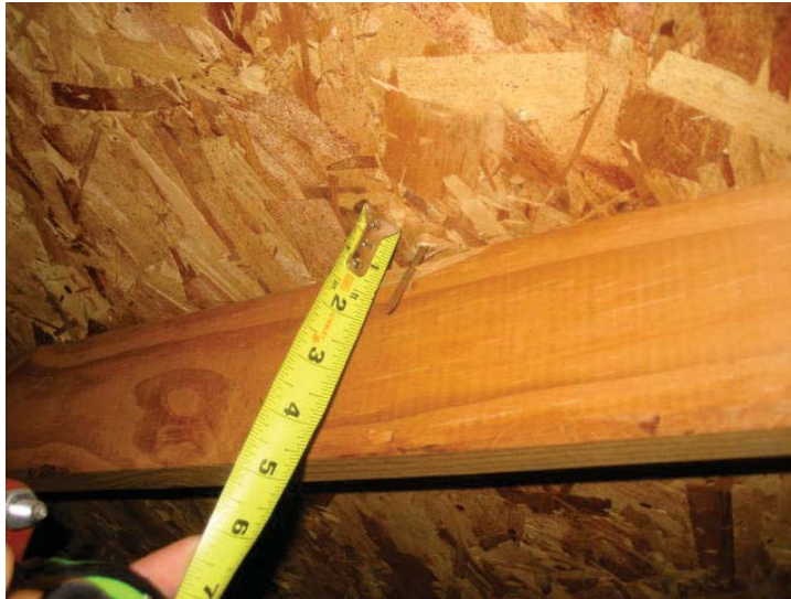
Roof Deck Attachment
