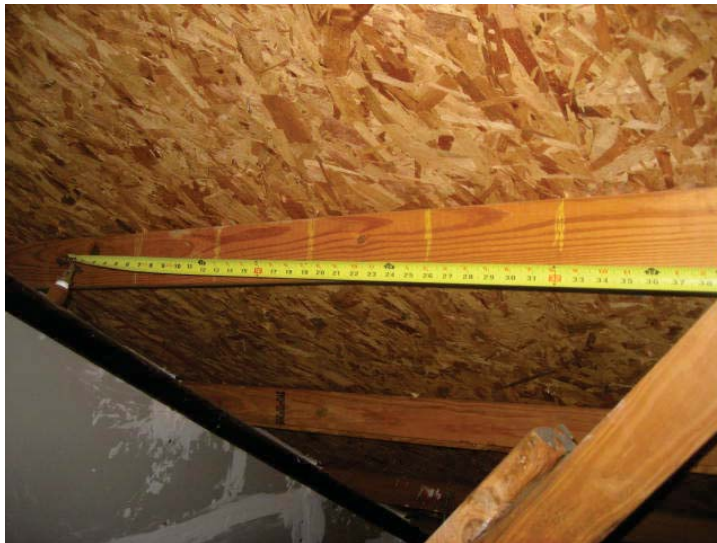
Roof Deck Attachment
